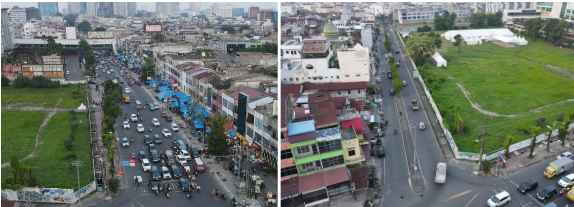
Figure 4. Road Conditions in the Study Area
